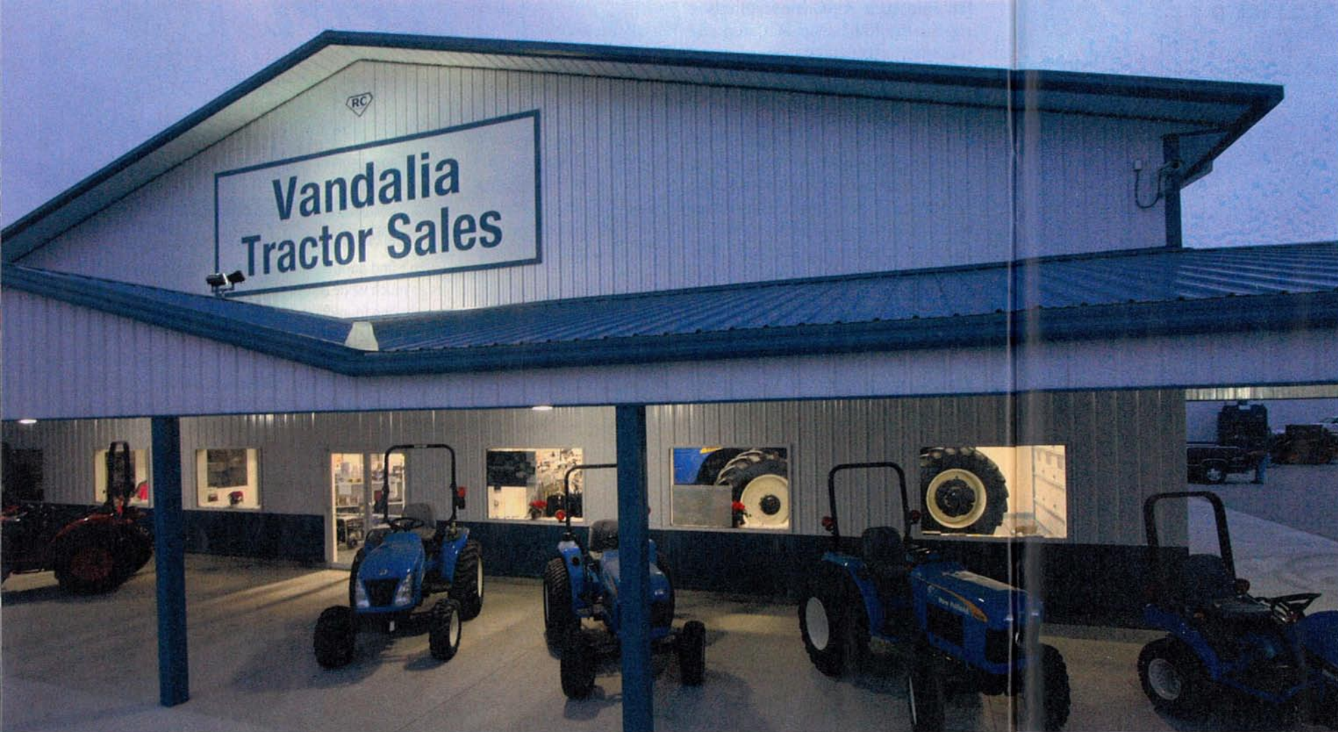
BUILDING A new facility from the ground up last year has paid dividends for Vandalia Tractor Sales in Vandalia, IL.
